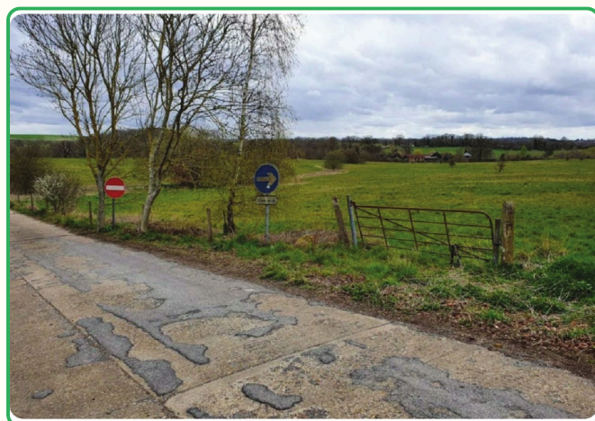
FRONTAGE FROM LOWER HATFIELD ROAD
