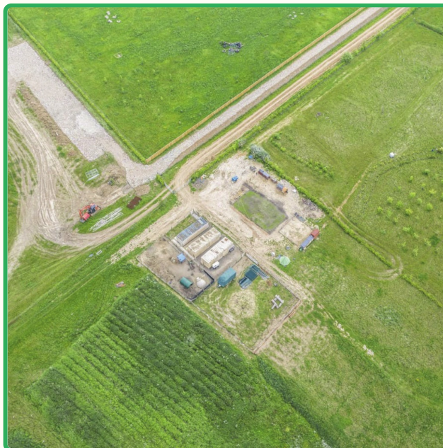
Site facilities & access track
