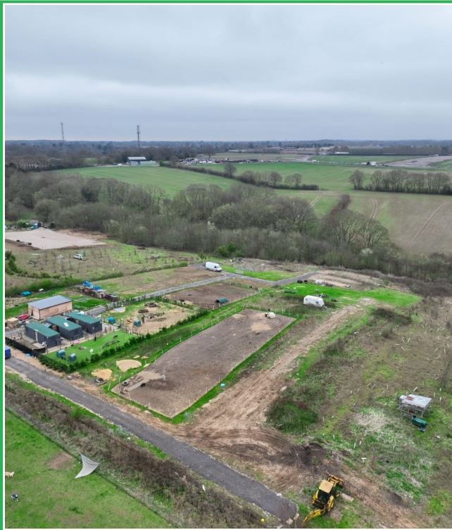
Aerial view — full site overview
