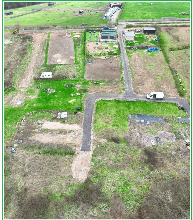
Aerial view — plots & access road
