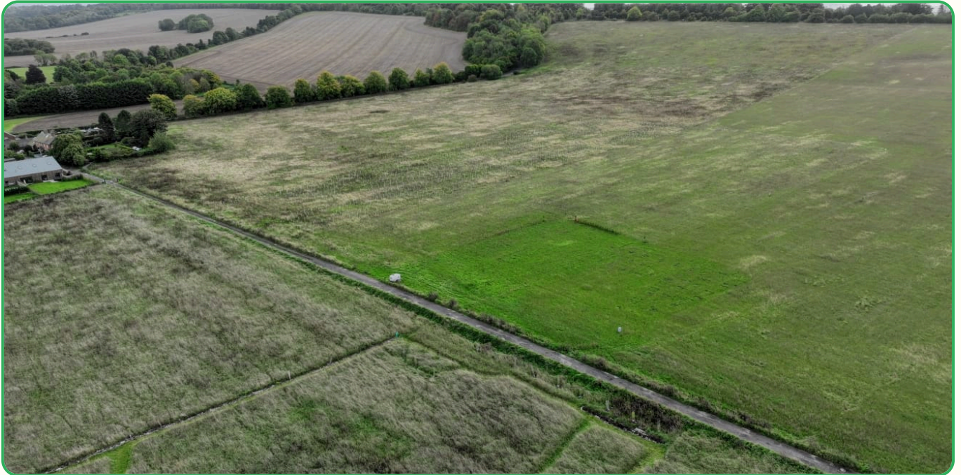
AERIAL OVER THE PLOT AREA AND THE PRIVATE ACCESS TRACK
