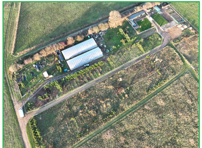
Aerial view — overhead site layout
