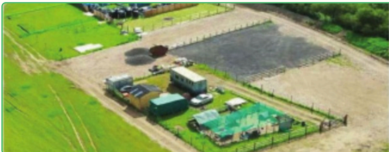
AERIAL VIEW OF THE HOLDING OFF WESTWOOD LANE
